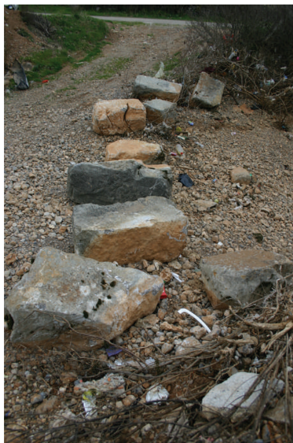
Sl. 8. Blokovi mosta, Vuksanlekići Fig. 8. Bridge blocks, Vuksanlekići
